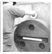
7. Wrap each seam with one wrap of 2" wide tape to bridge any possible gaps. **Note:** Tape not included. Finish installing concrete forms and pour concrete.
