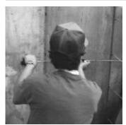
**1.** Locate center line where the hole is desired. This loca- tion will be used as a guide for the threaded centering assist rod.
