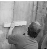
2. A 2x4 wood nailer is included. Fasten it along with the threaded rod directly to the concrete form. This provides support and helps center the complete Cell-Cast® disk assembly.
