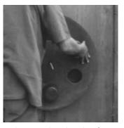
3. Slide the first Cell-Cast® disk over the \*threaded rod. Note: Use only 1 threaded rod for equal distribution. More than one rod could take disks out of shape.
