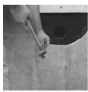
**9.** Chip excess concrete from the edge of the Cell-Cast® disk assembly and wall.
