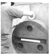
7. Wrap each seam with one wrap of 2" wide tape to bridge any possible gaps. **Note:** Tape not included. Finish installing concrete forms and pour concrete.
