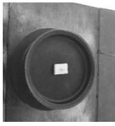
Place second cap on the sleeve and use a (block of wood\*) and (wing nut\*) to tighten unit in place. Make certain sleeve is plumb.
