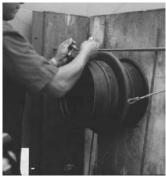
5. For additional stability, it's necessary to secure the sleeve with wire to the rebar. Insert the other end cap firmly, check that second end cap is positioned correctly, confirm sleeve length and close the form.
