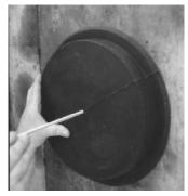
After nailing end cap to form, drive (threaded rod\*) through the end plate and form and (thread nut\*) on other side.
